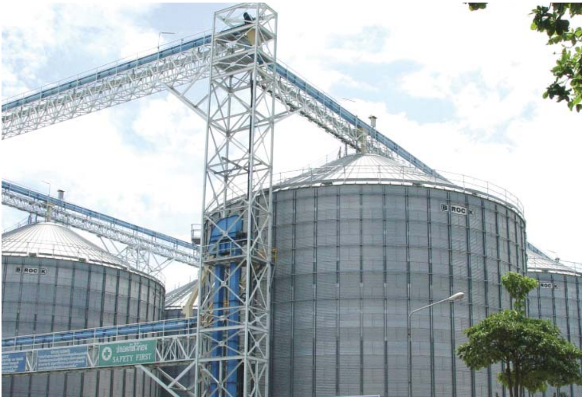
One of Betagro's newly completed feed mills.
